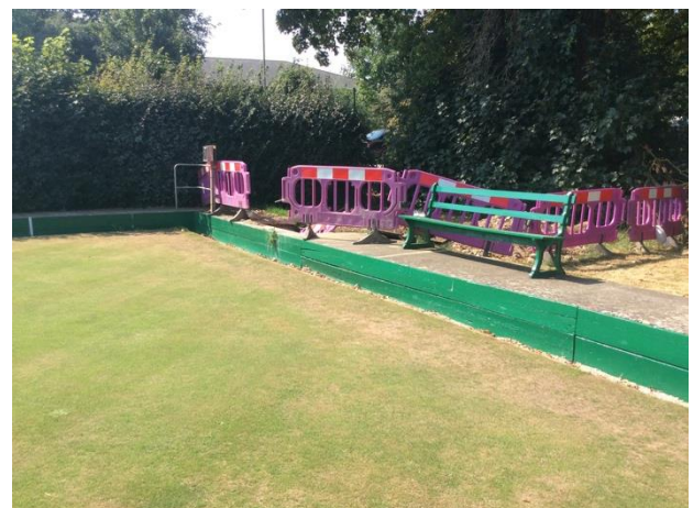
Figure 18: Some groundworks have been undertaken on the utilities traversing the site and it is not known if this may have impacted the irrigation system leading to the problems currently faced.
